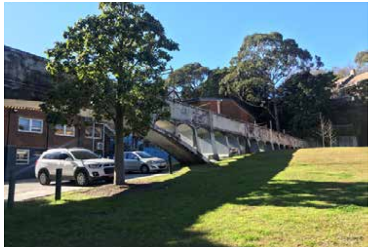
View to Johnsons Creek Aqueduct
